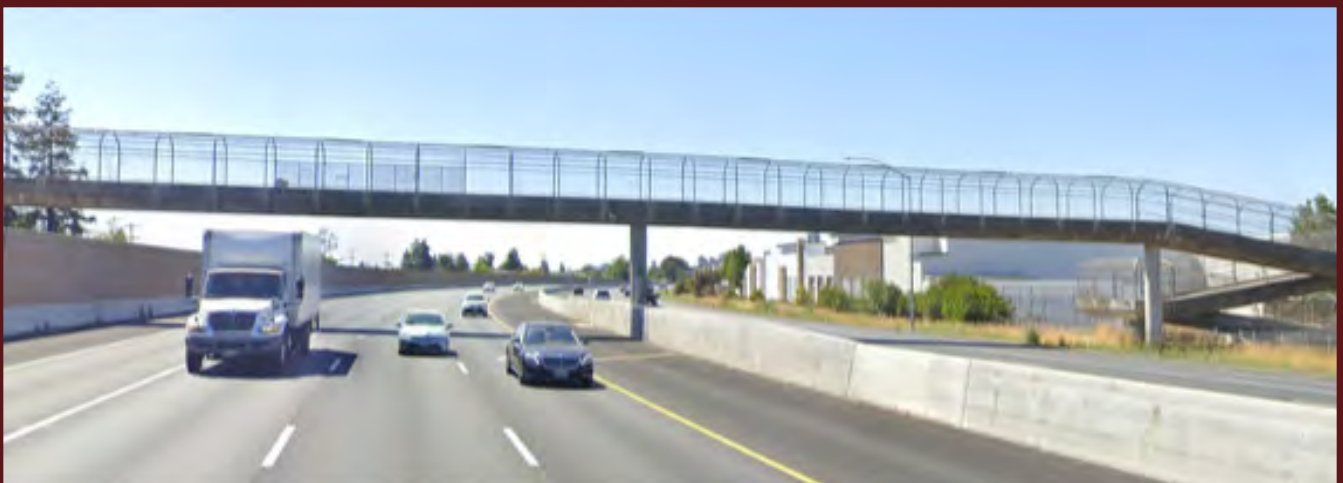
Figure 4.18 Example Active Transportation Grade-Separated Highway Crossing
