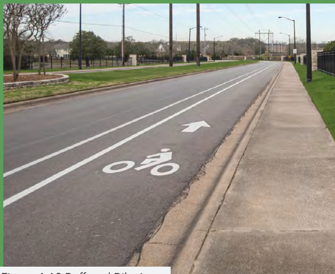
Figure 1.10 Buffered Bike Lane
