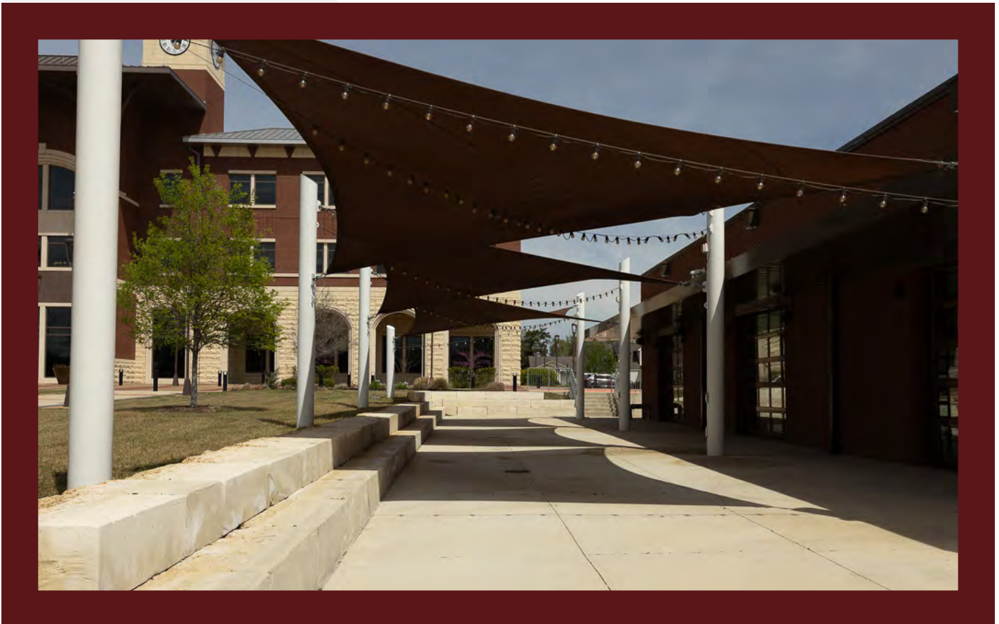
Figure 4.16 City Hall Structured Shading
