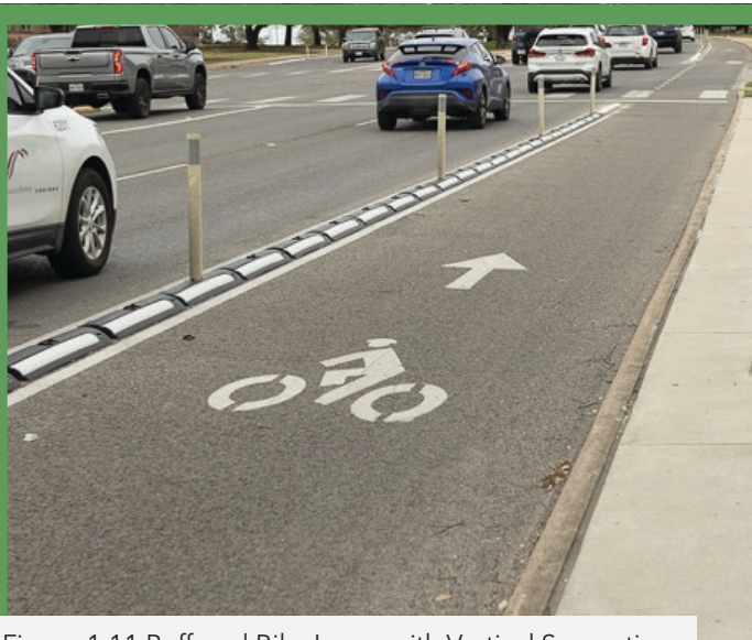
Figure 1.11 Buffered Bike Lanes with Vertical Separation
