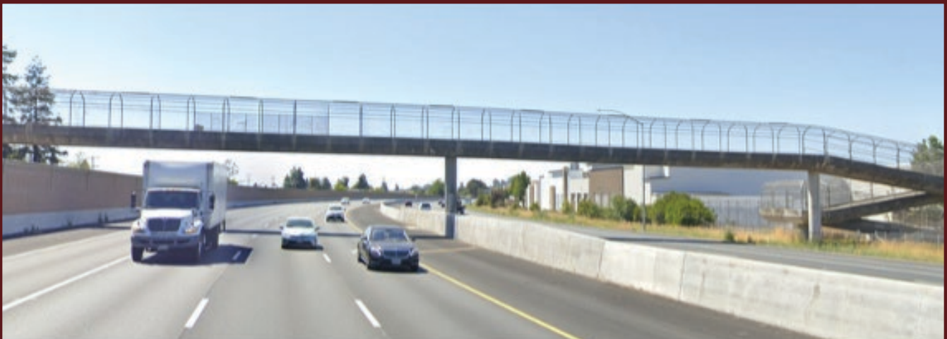
Figure 4.18 Example Active Transportation Grade-Separated Highway Crossing
