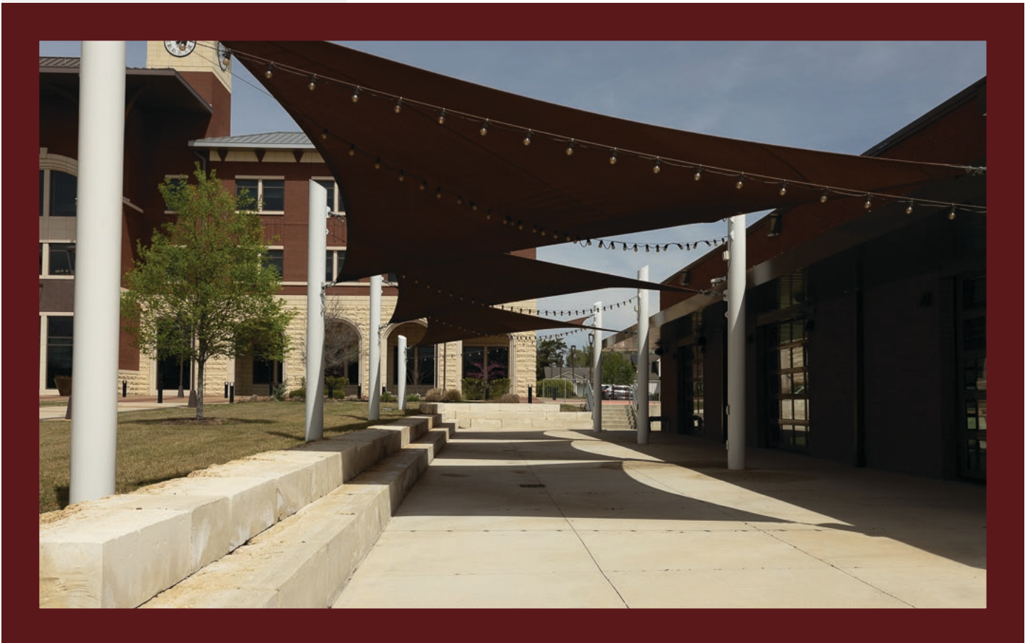
Figure 4.16 City Hall Structured Shading
