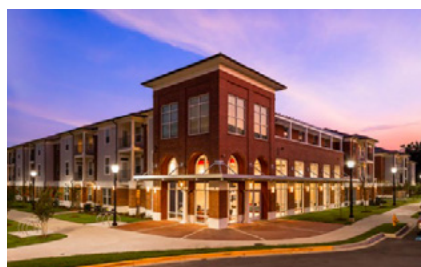
The Heritage at Cajun Village Lafayette, Louisiana
